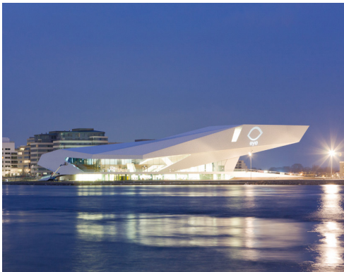
The EYE Film Institute Netherlands relies on top-quality projection equipment from Kinoton
